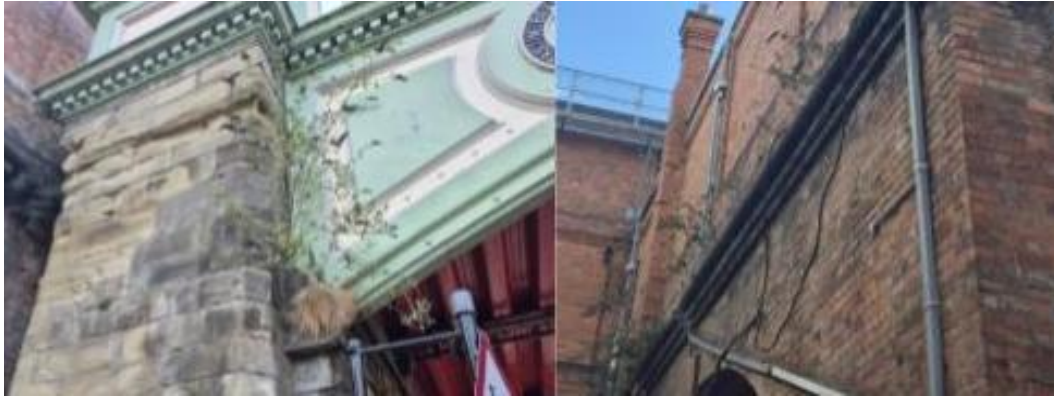
Buddleia in high-level brickwork, Worcester Foregate Street Station
