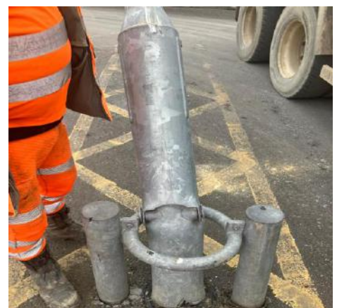
Lighting column damaged
