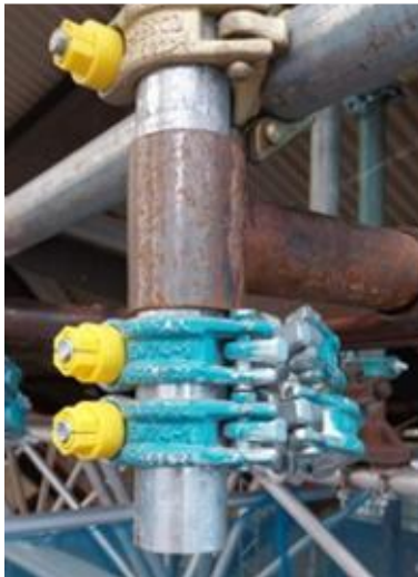
Revised detail with swivel coupler fittings permitting visual inspection of both fittings by erector. Note: Yellow Clikon caps to aid inspection.
