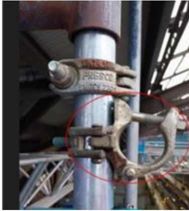
Bottom fitting was acting as supplementary coupler. Note: Not the actual fitting, this is a similar arrangement.
